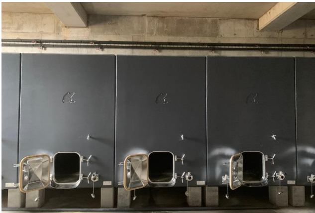
Concrete boxes for the "White Label - APS Cuvée"
